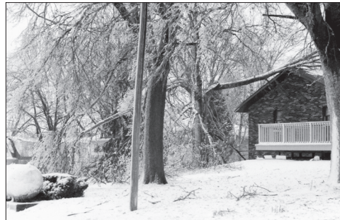
A huge tree split in two falling with a crash onto the roof of Pastor and Barb Gorter's house.
