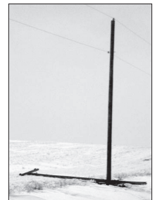
Poles cracked off causing power outages until crews arrived to replace them.
