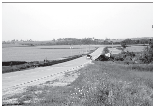
The river bottom flooded, closing roads and turning part of Richland Township into two giant, but scenic lakes for a brief period of time. Top: Some of the water even lapped at the buildings on Keith Van Ee's farm.
