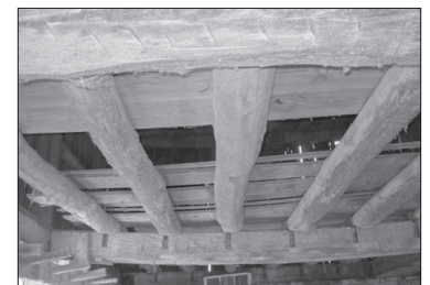
Spaced logs allowed for hay mow air circulation.
