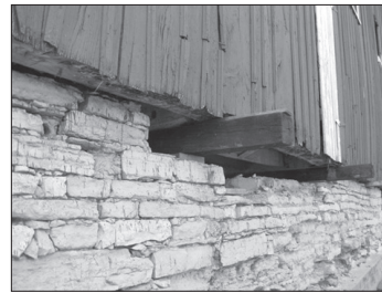
The foundation is still doing its job after 150 years.
