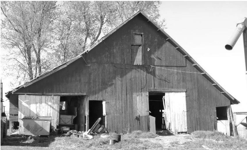
The old red barn on the Vos property, there were two leans on the barn that were compromising the structure that needed to be removed
