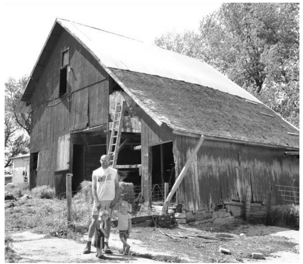
The old red barn on the Vos property, there were two leans on the barn that were compromising the structure that needed to be removed
